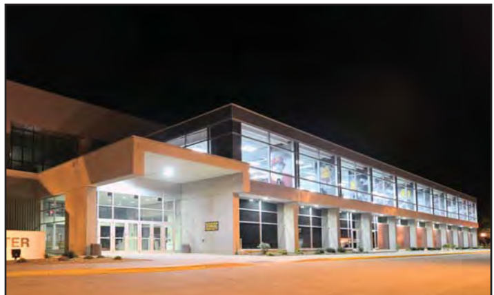
Barnett Center Addition - Aberdeen, SD
