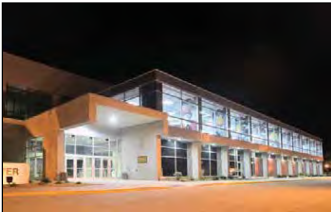
Barnett Center Addition - Aberdeen, SD
