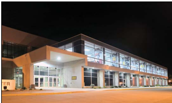
Barnett Center Addition - Aberdeen, SD
