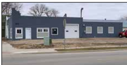
PA Towing 317 1st Ave SE Exterior Improvements
