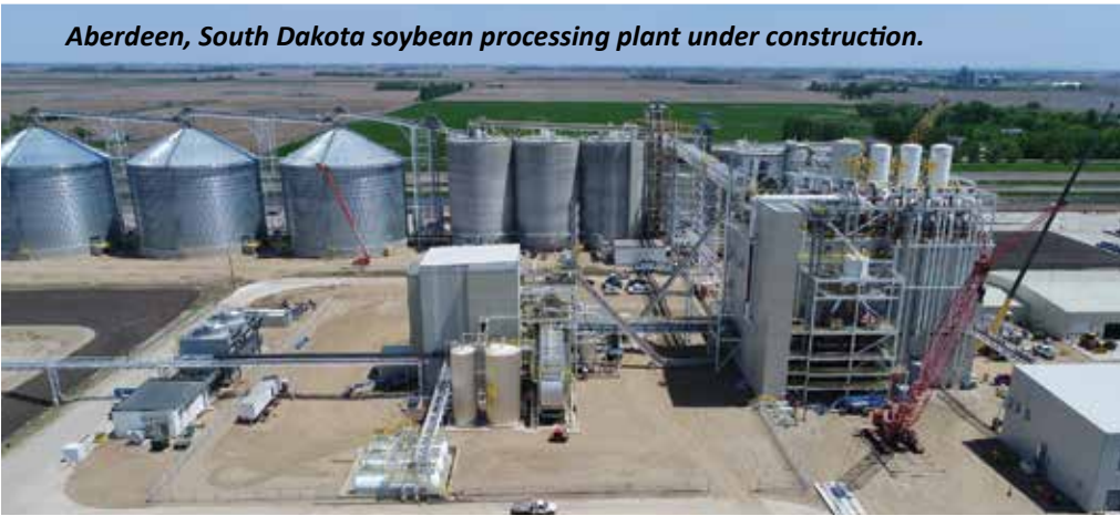
Aberdeen, South Dakota soybean processing plant under construction.
