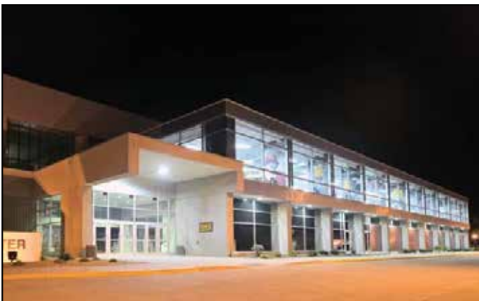
Barnett Center Addition - Aberdeen, SD
