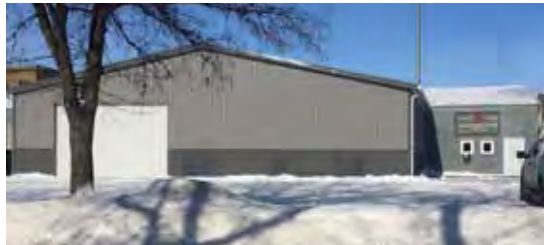
Forsyth & Zahn Construction
