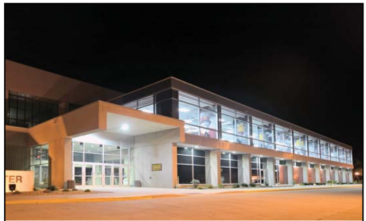
Barnett Center Addition - Aberdeen, SD
