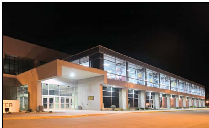
Barnett Center Addition - Aberdeen, SD
