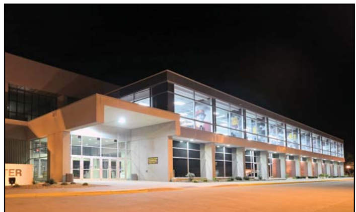
Barnett Center Addition - Aberdeen, SD
