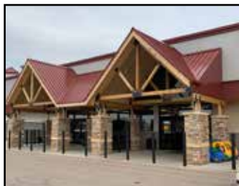
Ken's Super Fair Foods 2105 6th Ave SE Exterior improvements
