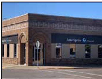
Ameriprise Financial Services 101 3rd Ave SW Exterior improvements
