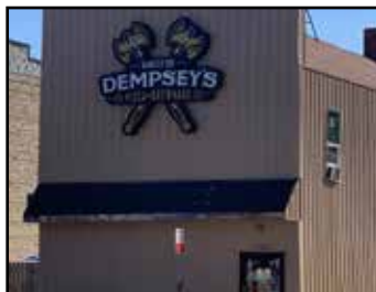
Danger von Dempsey's Pizza & Brewhaus 1023 S Main St Exterior improvements
