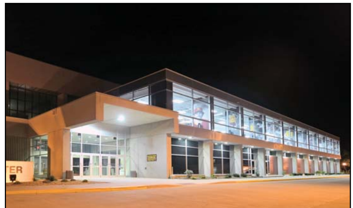
Barnett Center Addition - Aberdeen, SD
